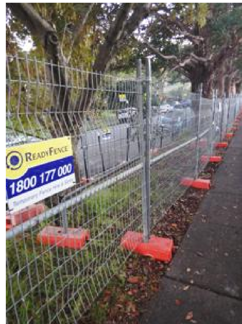
Example image of acceptable tree protection fencing measures to be applied. (1.8m high rigid metal fencing with appropriate lateral bracing)
