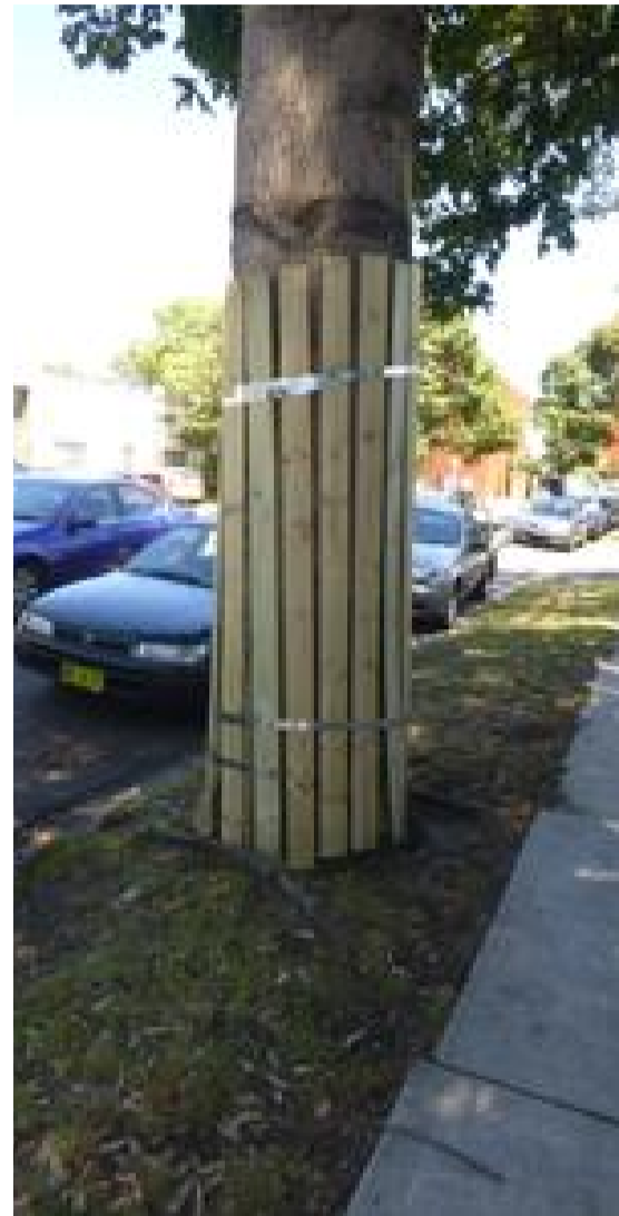
Example image of acceptable tree protection battens
